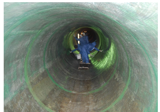
Figure 7(d): Detailing of FRP lining
