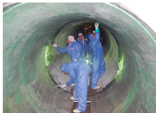
Figure 7(a): Epoxy paste installation on top half of pipeline
