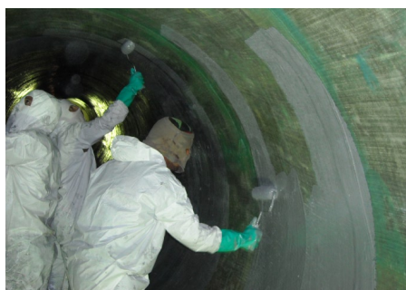
Figure 9: Application of epoxy top coat
