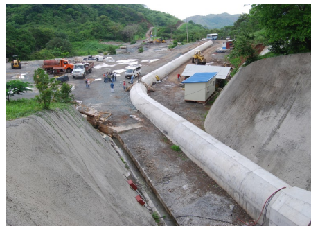
Figure 1: Above ground segment of the "El Encanto" pipeline
