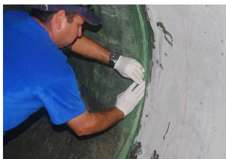
Figure 8: Construction joint of FRP lining
