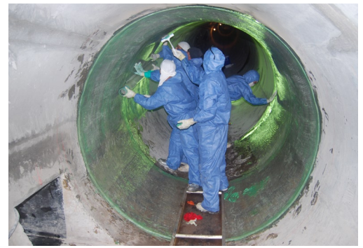
Figure 7(b): Installation of FRP lining
