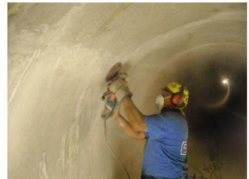
Figure 5: Prep work activities prior to installing FRP lining
