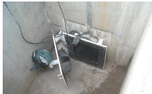
Figure 6: Typical 2 ft. x 2 ft. access point
